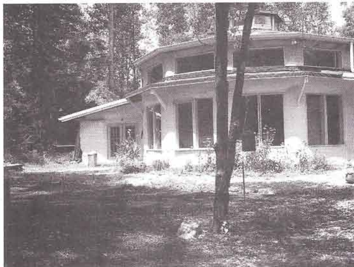
The Council Hall at Earthaven supports meetings and was once (during a very difficult period) the office of the Permaculture Activist.
